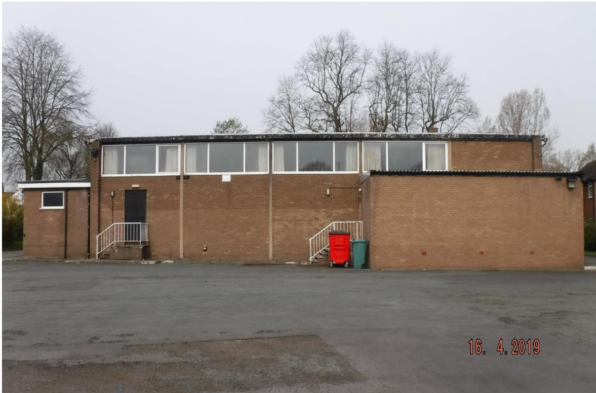
Photograph 2. Car park and east aspect of the building.
