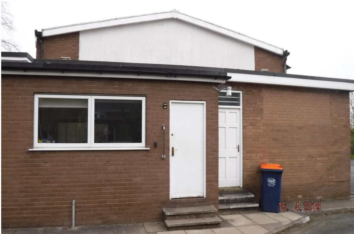
Photograph 4. South aspect of the building with pitched roof visible.
